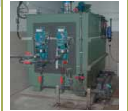
Reagent pumping - polymer injection - lime milk pumping - transfer of activated charcoal
