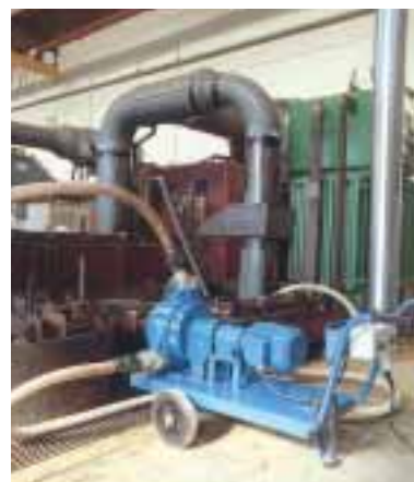
Z pump in draining of wells
